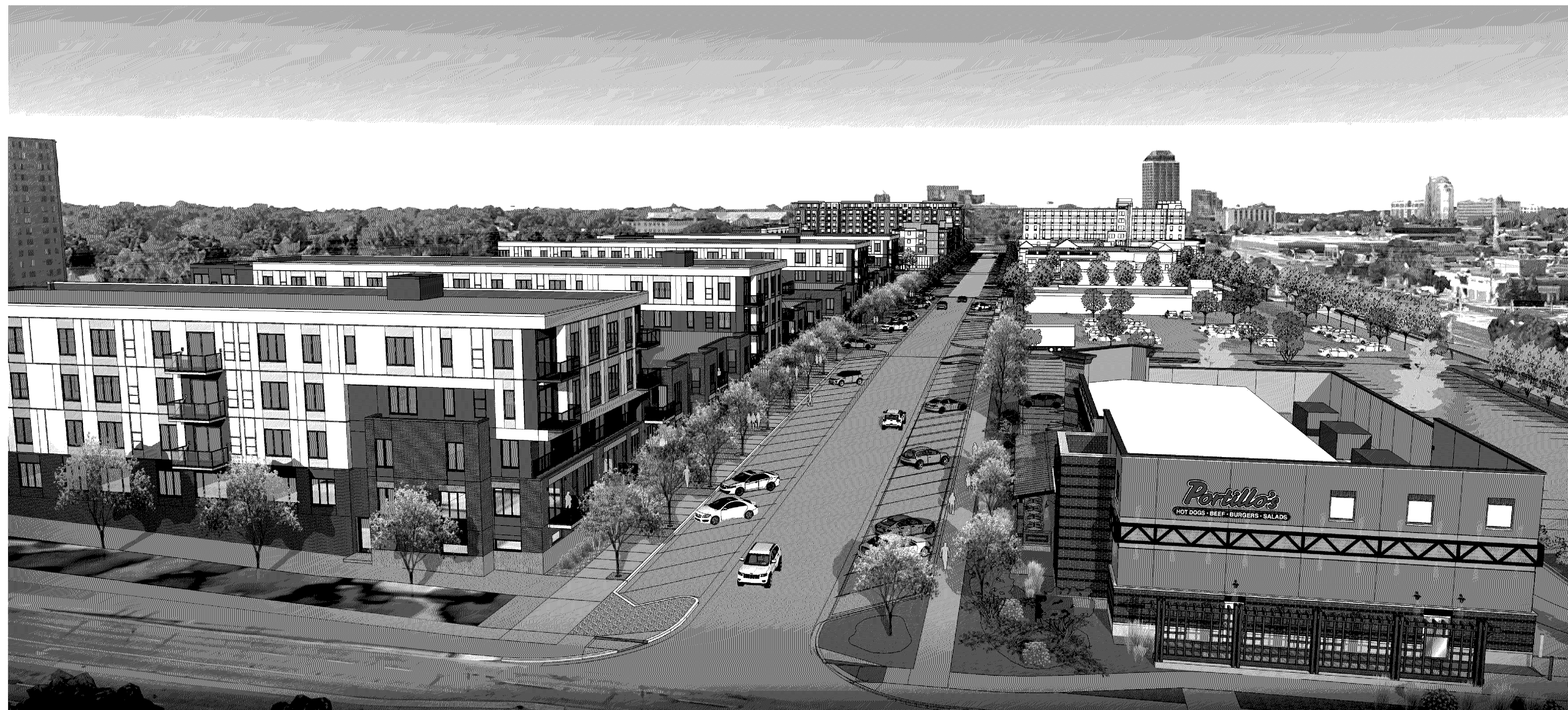
BIRDSEYE VIEW OF LOOKING WEST DOWN 80-1/2 STREET
