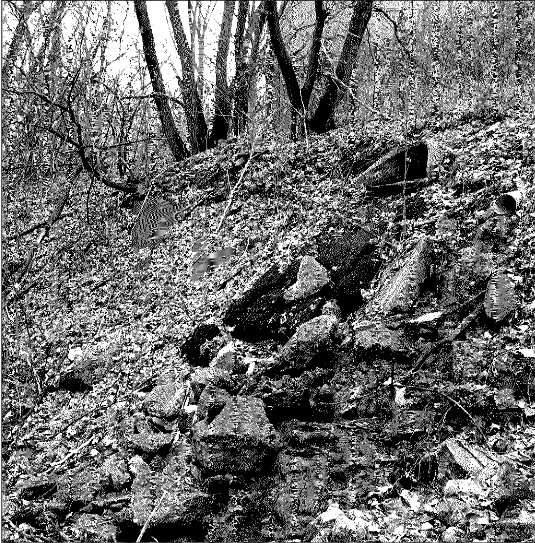
Photograph 10. West Slope of Pond
