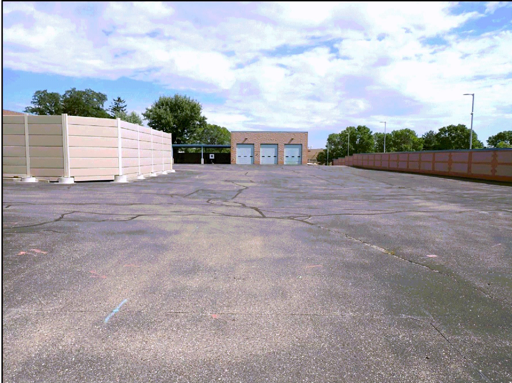
1 EXISTING PHOTO SCALE: NONE
