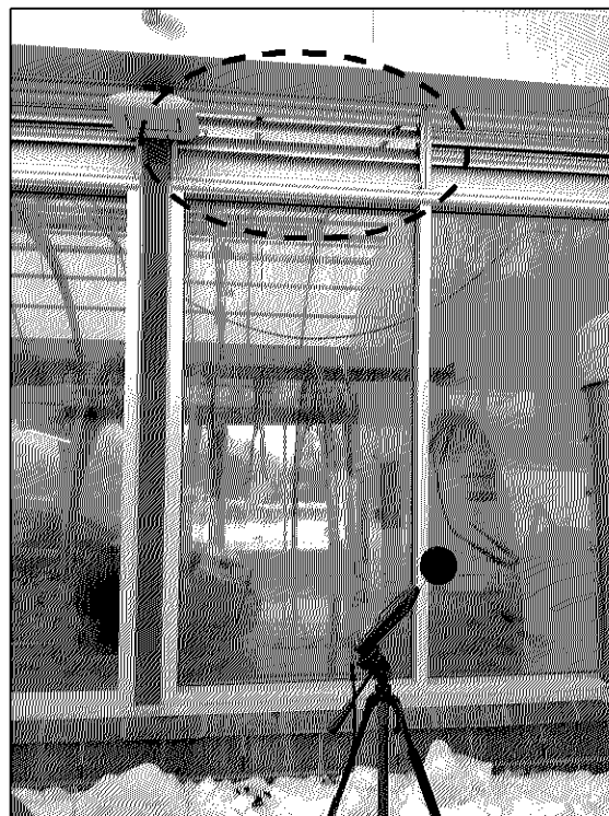
Figure 8 – Photo of the Tommy's Express Car Wash with an open damper circled.
