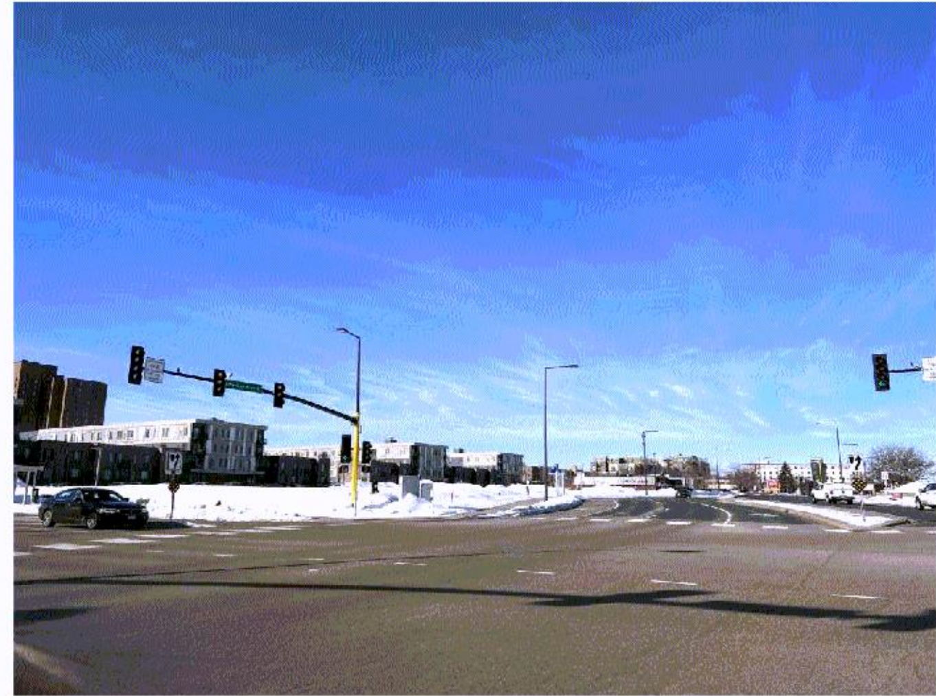
SITE PHOTO: VIEW SOUTHWEST TOWARD SITE
