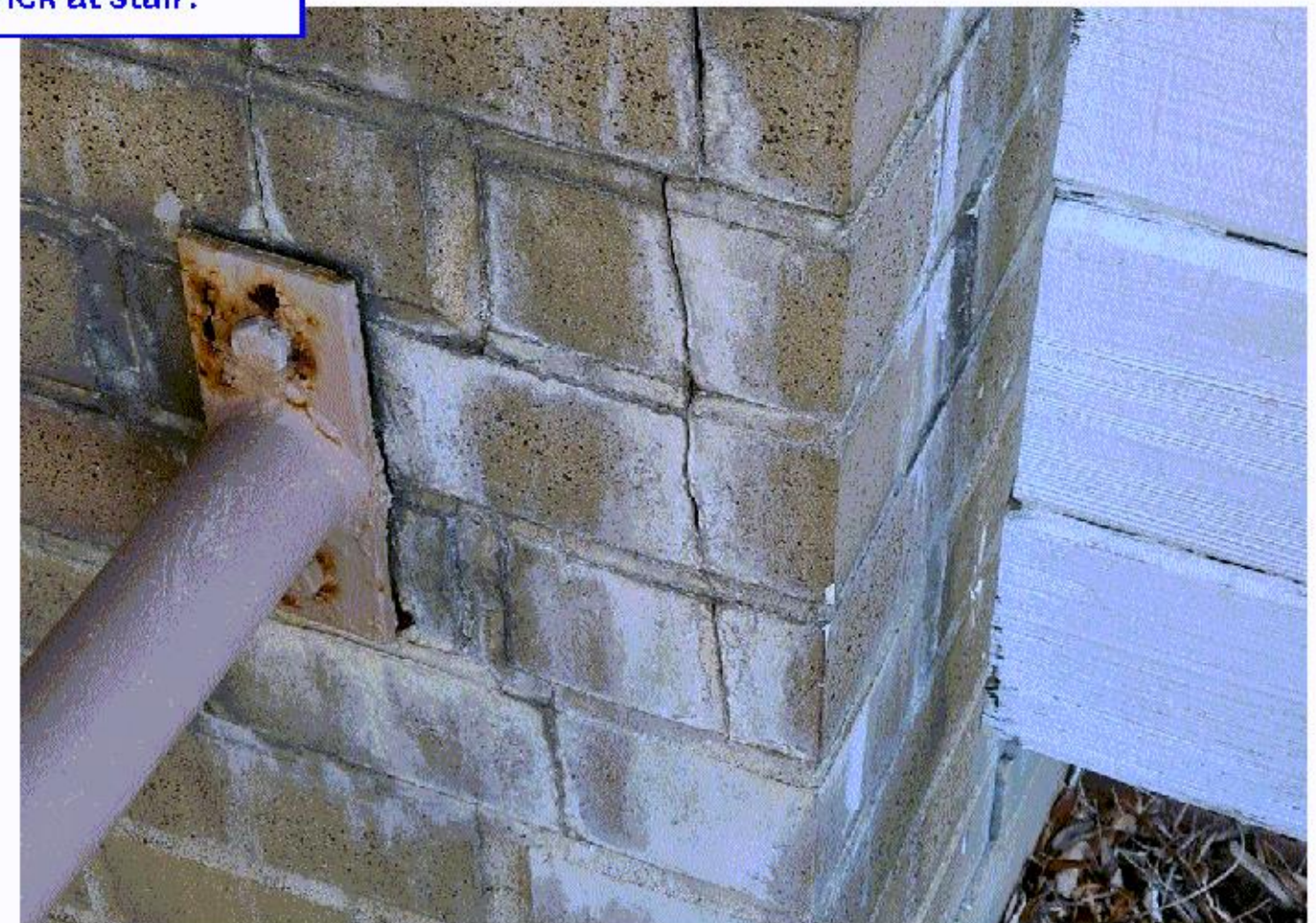
G: Repair eroded block at corner and grout brick at stair.
