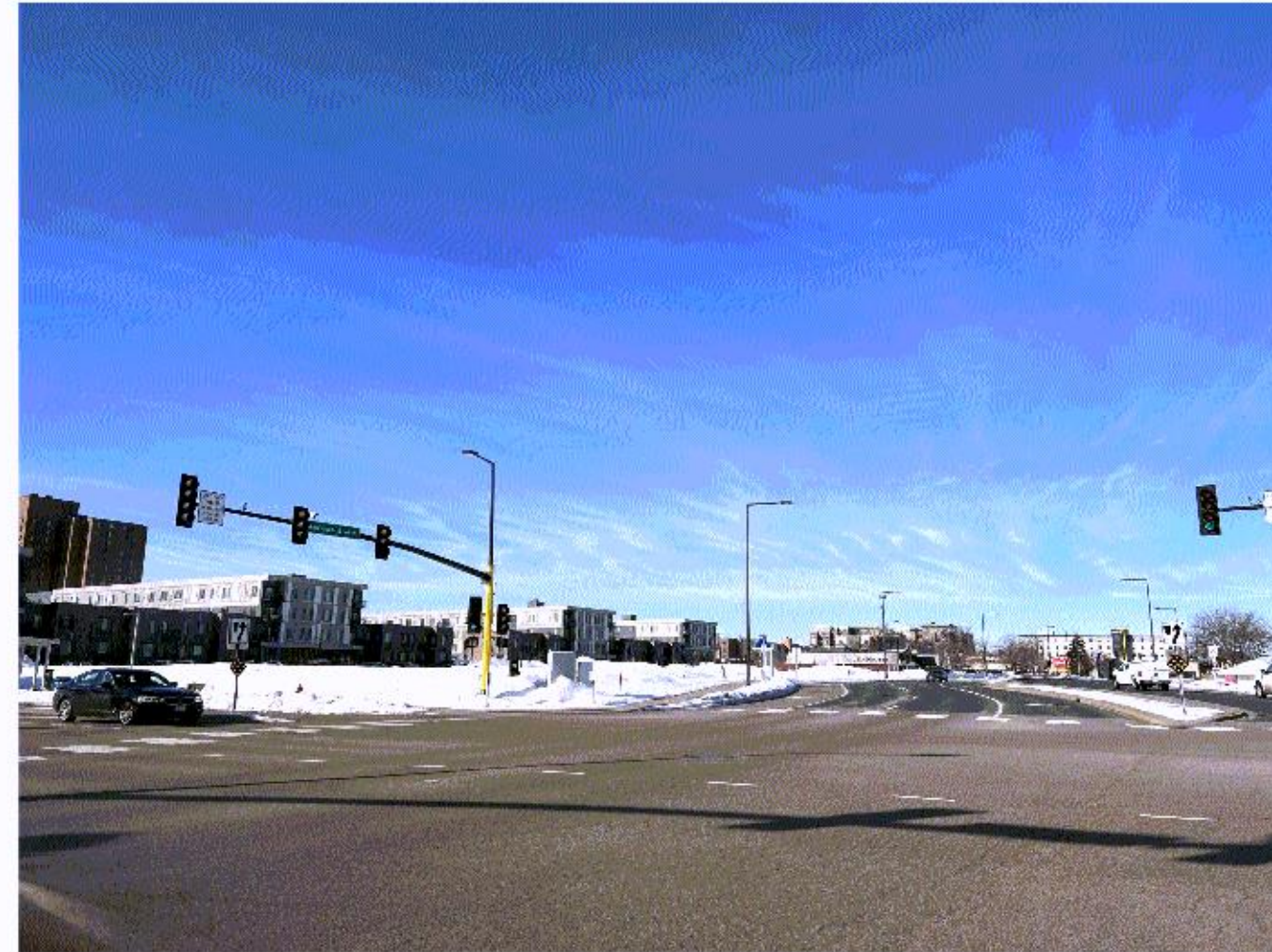
SITE PHOTO: VIEW SOUTHWEST TOWARD SITE
