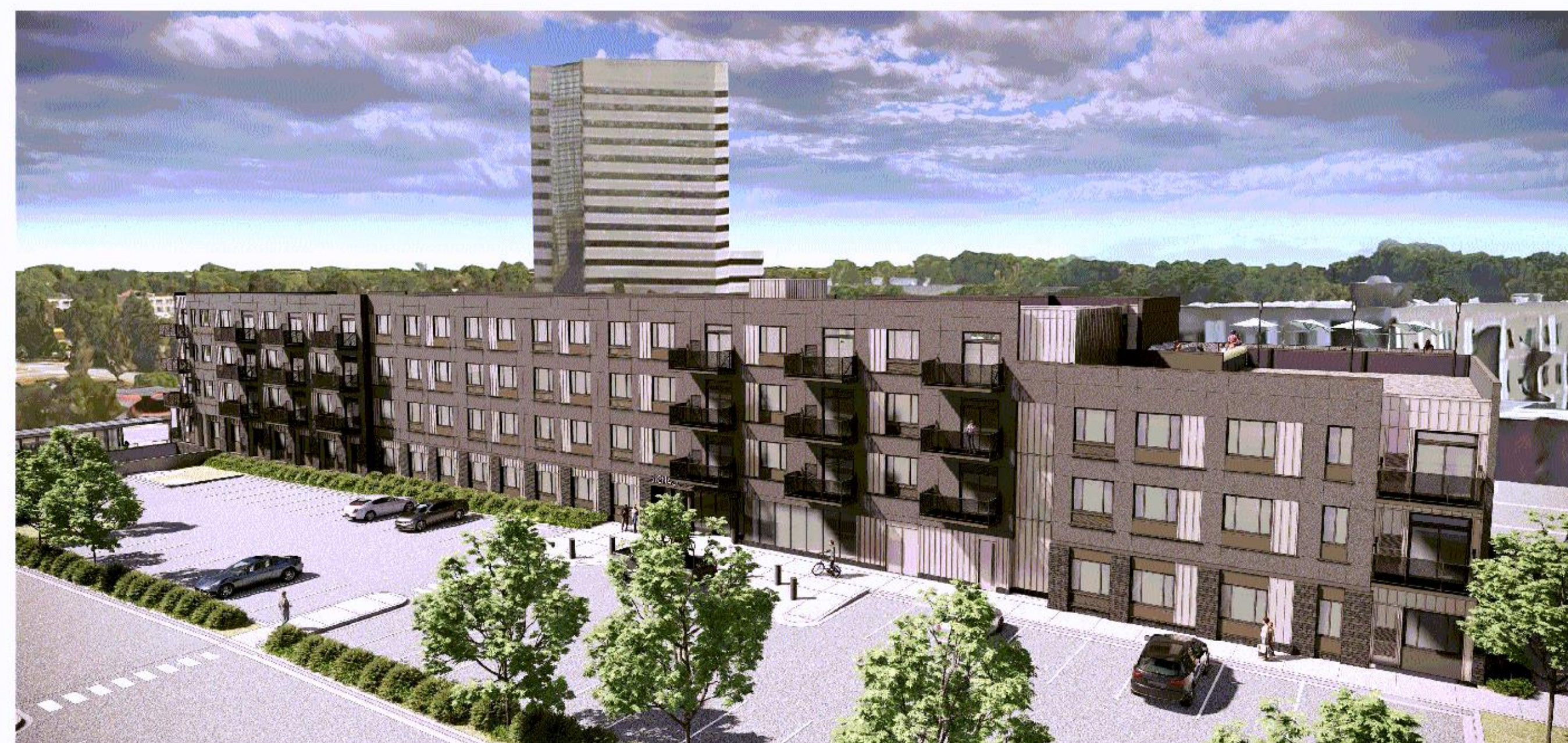
VIEW OF NORTH ELEVATION LOOKING SOUTHEAST
