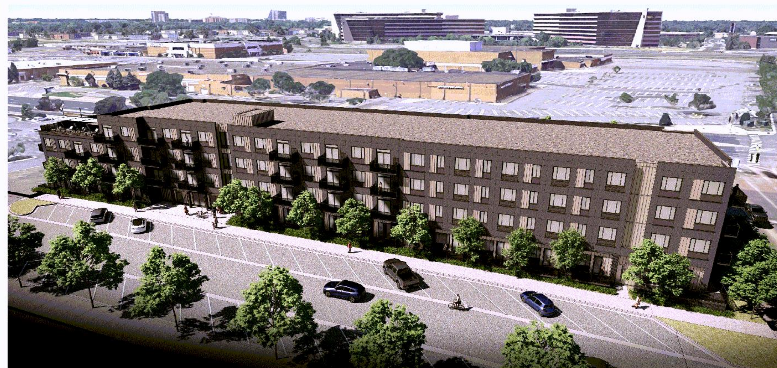
AERIAL VIEW OF 80-1/2 STREET FRONTAGE LOOKING NORTH
