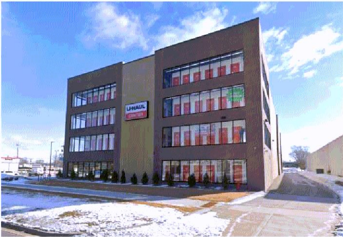
U-Haul Self Storage Facility 8901 Lyndale Ave 4 stories, 103,984 square feet (included CUP for self-storage use)
