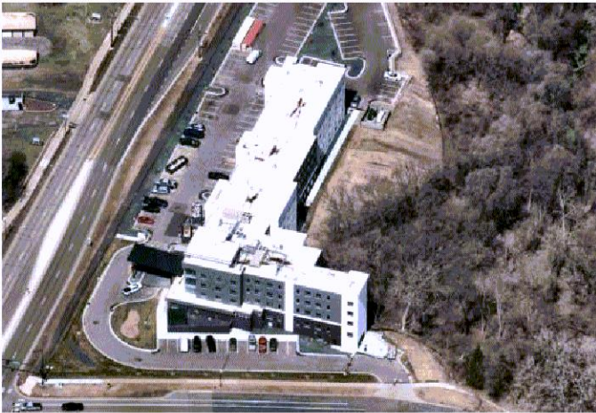
Hyatt House Hotel 2301 E Old Shakopee Rd Four story, 151-rooms, 98,744 square feet
