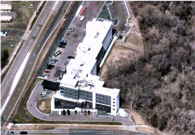
Hyatt House Hotel 2301 E Old Shakopee Rd Four story, 151-rooms, 98,744 square feet
