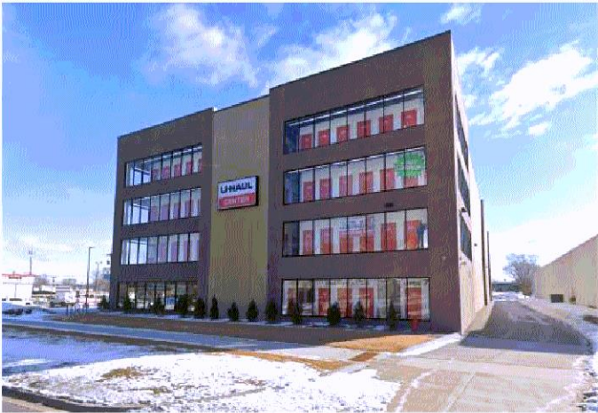
U-Haul Self Storage Facility 8901 Lyndale Ave 4 stories, 103,984 square feet (included CUP for self-storage use)
