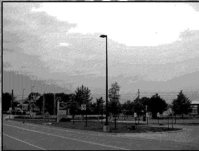
B SITE OVERVIEW [LOOKING NORTHWEST]
