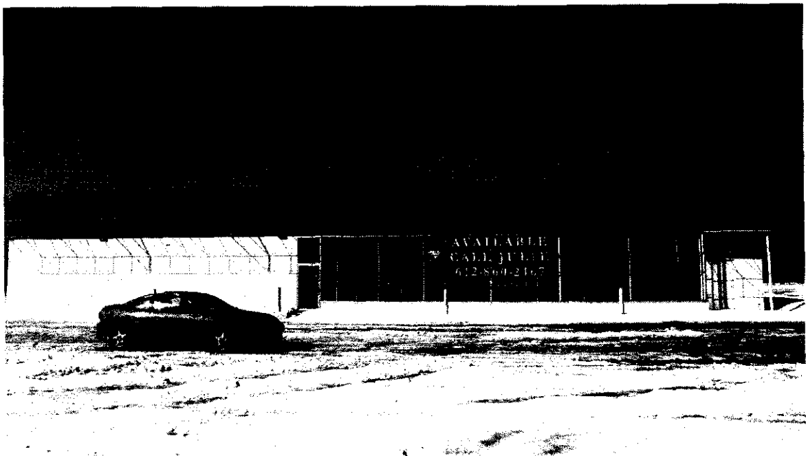
Existing front (east) facade
