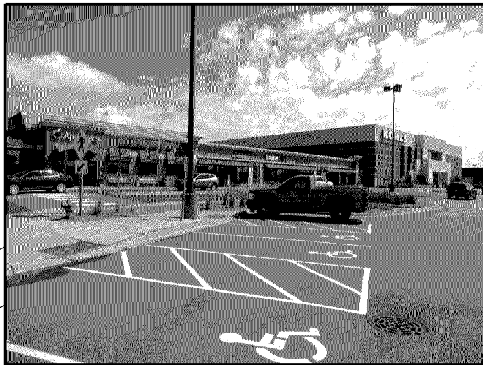
SITE OVERVIEW [LOOKING NORTHEAST]
