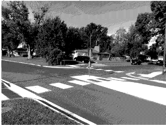
Intersection Improvements (Park Ave & E 82 nd St)
