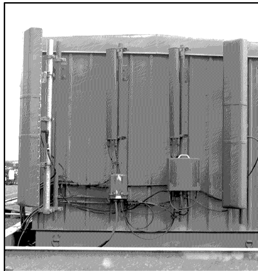
4 'X' SECTOR ANTENNA MOUNT PHOTO SCALE: NONE
