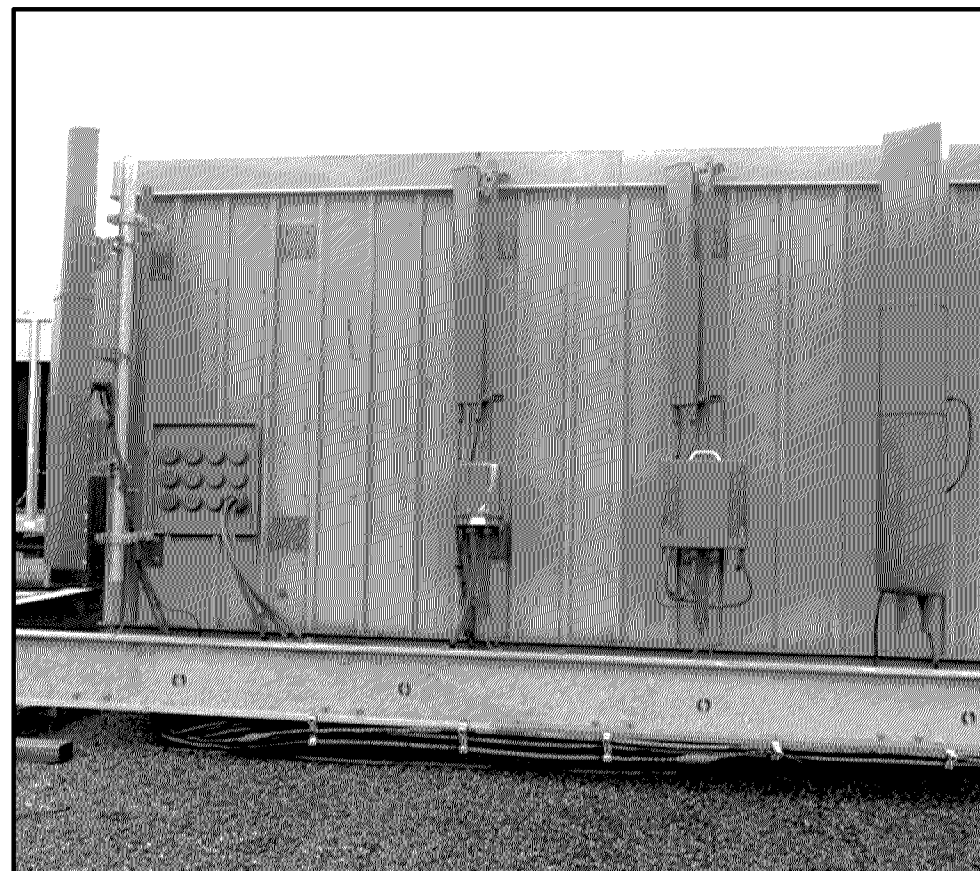
5 'Y' SECTOR ANTENNA MOUNT PHOTO SCALE: NONE
