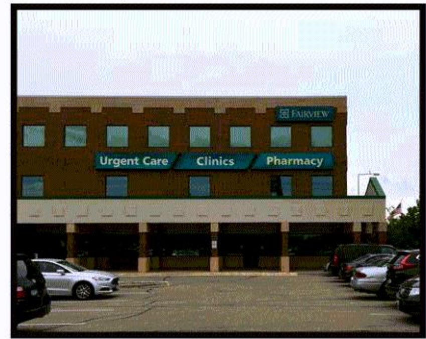
Existing West Elevation (4) Cabinets to be Removed
