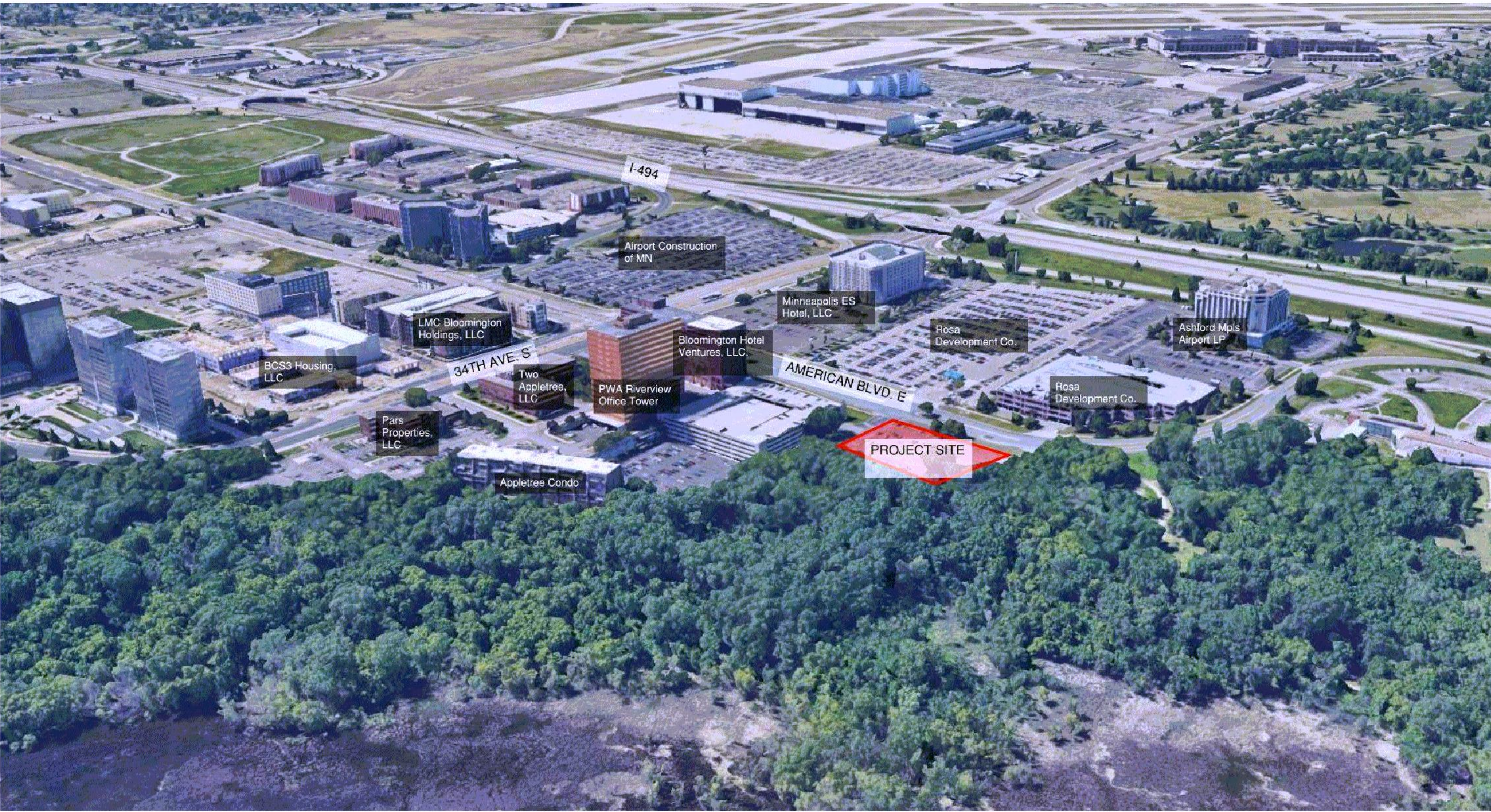
PROJECT AERIAL VIEW WITH ADJACENT PROPERTY OWNERS
