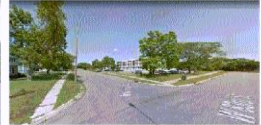
Existing Street View - Irving Ave & B3rd St
