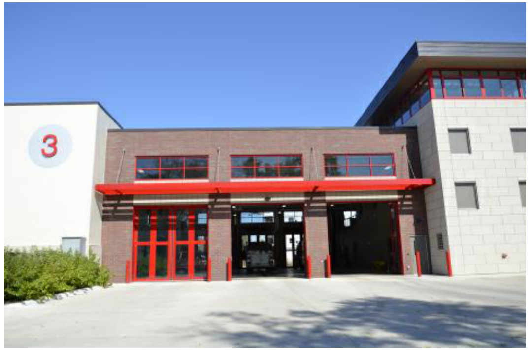
BLOOMINGTON FIRE STATION 3 2301 E 86TH STREET BLOOMINGTON, MN 55425
